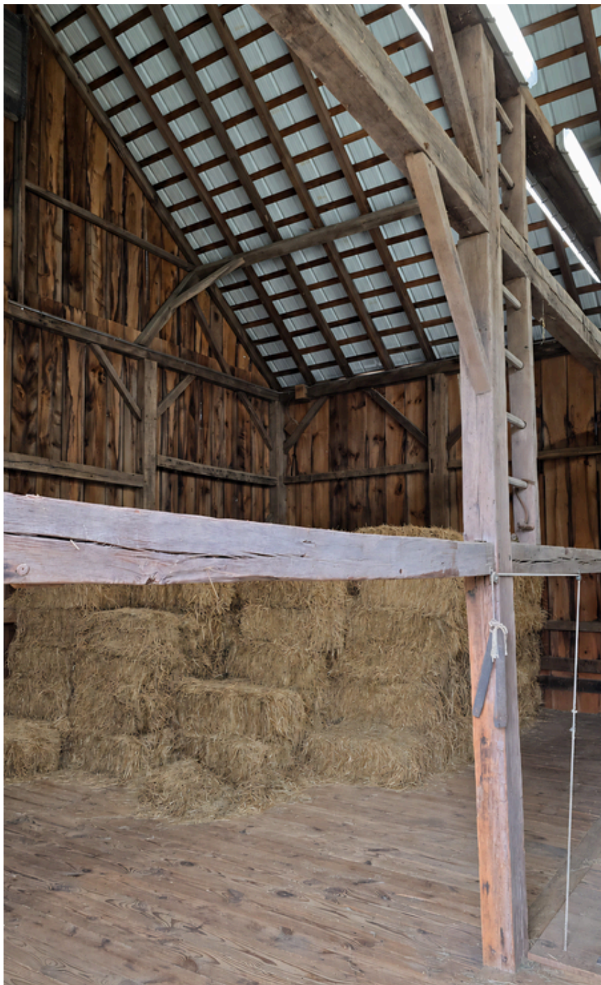
Original hand-hewn oak posts and beams in the hayloft.
