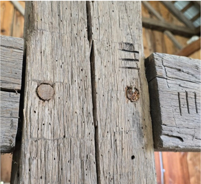
Beams were marked for reassembly, and pegs were reused where possible.
