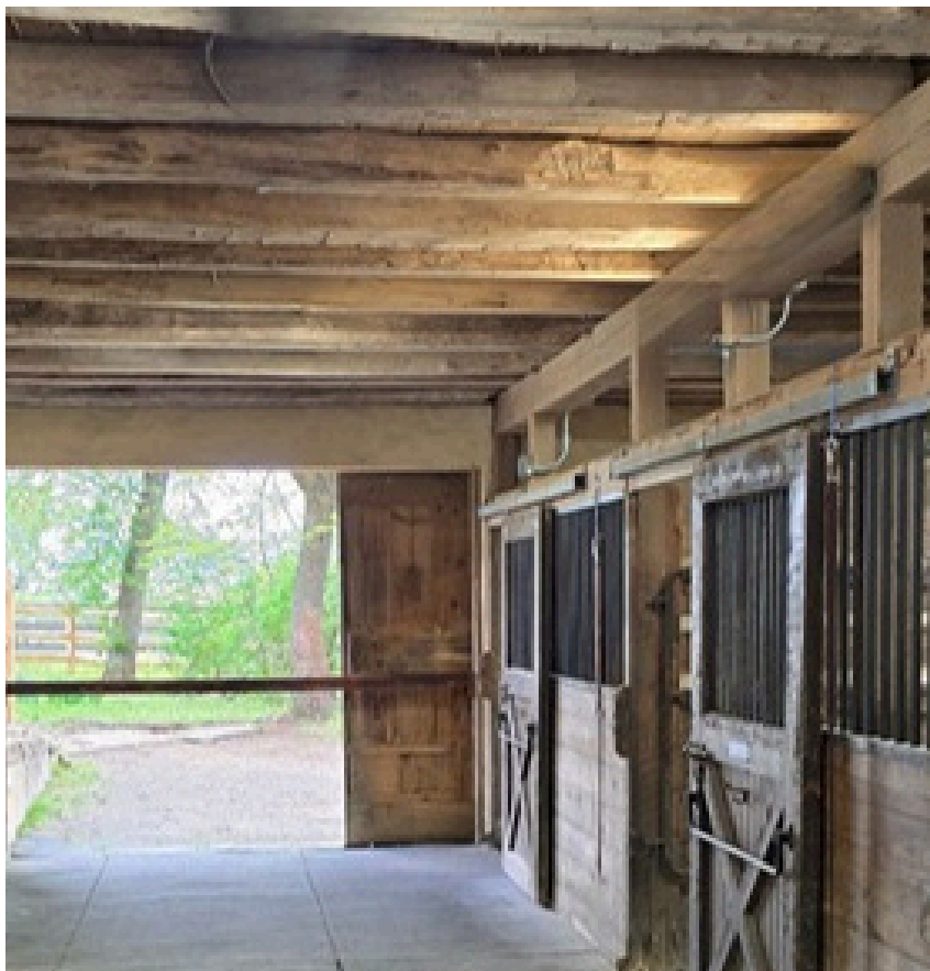
Tack/feed room and horse stalls in the lower level of the barn.
