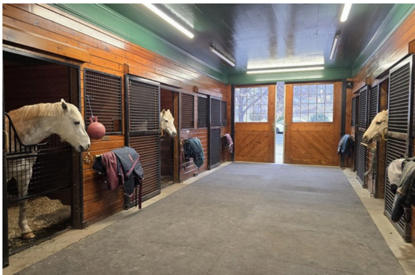
Metal stall gates give good ventilation and allow the horses to visit in the aisle.
