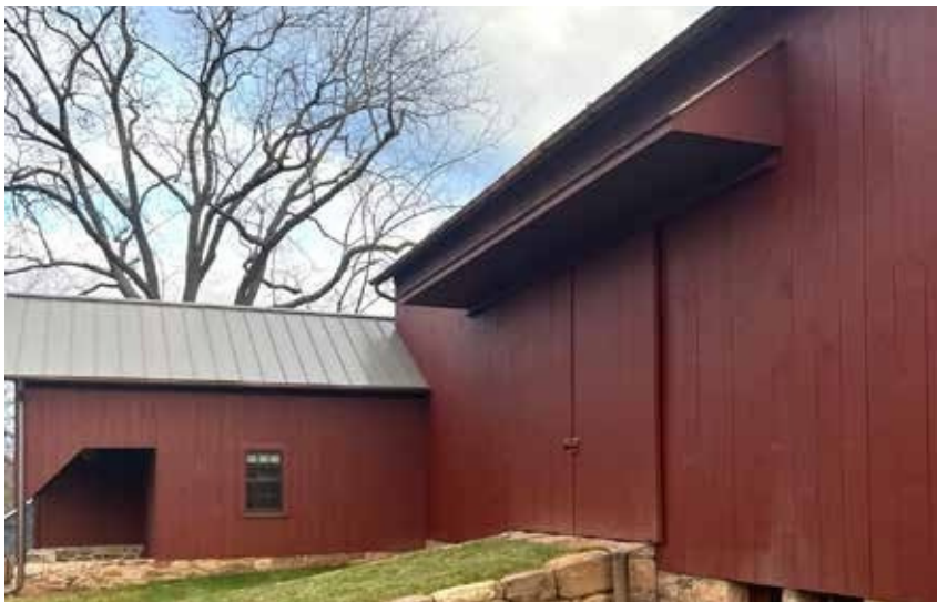
An exterior view of the main barn facing north with the bank access to the upper level.
