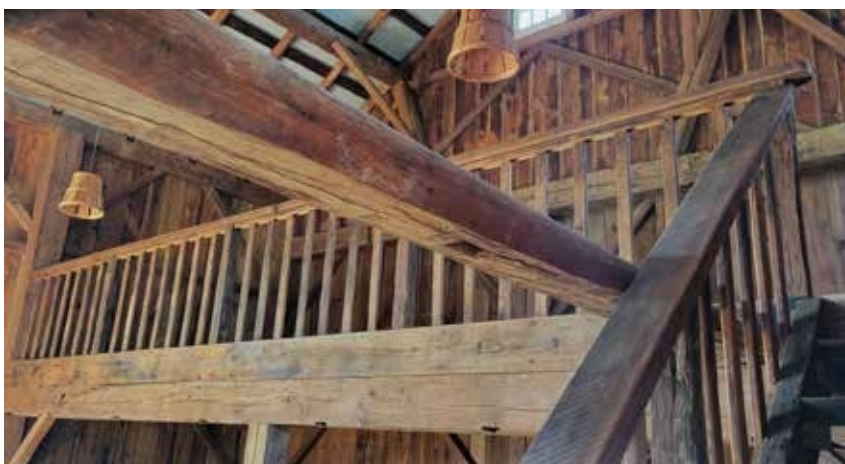
An interior view of the main barn looking at the west end loft.
