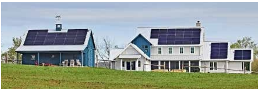
Glenn Wheat in Spring. Solar panels generate 5 megawatts more than we use each year.
