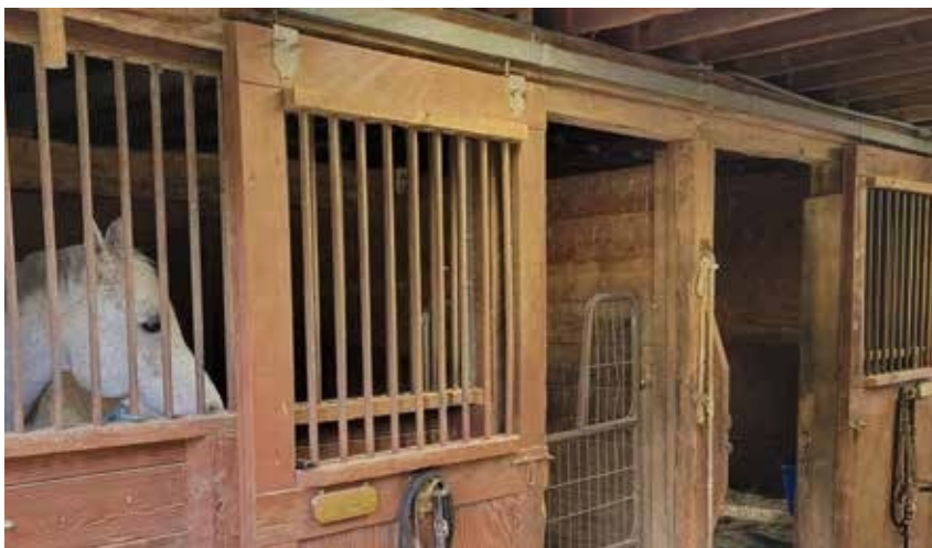
The older barn has a post and beam construction.
