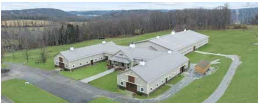
A view of the main barn at the top of Hart Farm.
