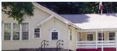
60 Water Street, Mountainville
